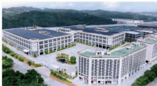
SHUA Industrial Park in Quanzhou Taiwan Investment Zone (Unit 2)
