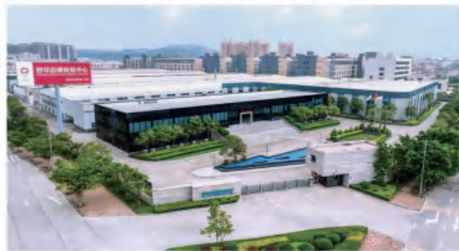
SHUA Industrial Park in Quanzhou Taiwan Investment Zone (Unit 1)
